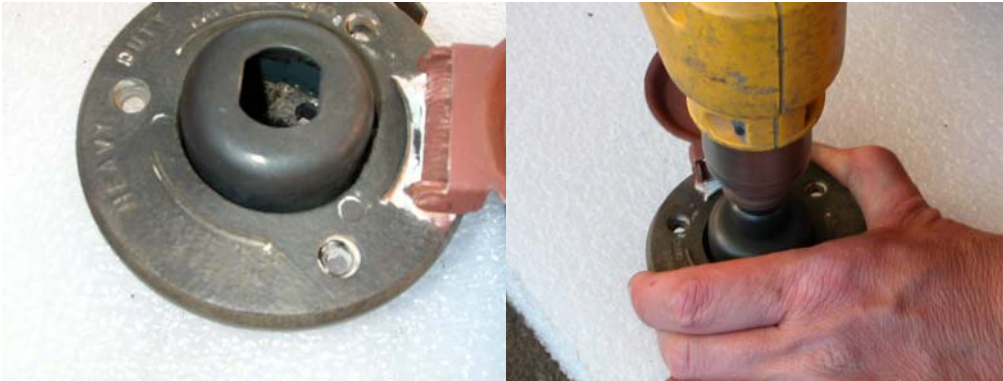
Fit of hole saw
