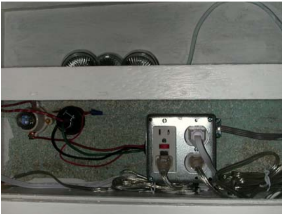
Plug installed w/ quad GFCI box just after
